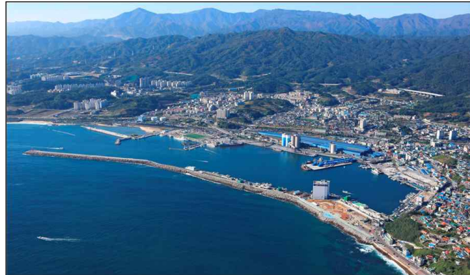
Fig. 2.7 The present status of port redevelopment sites (2)
