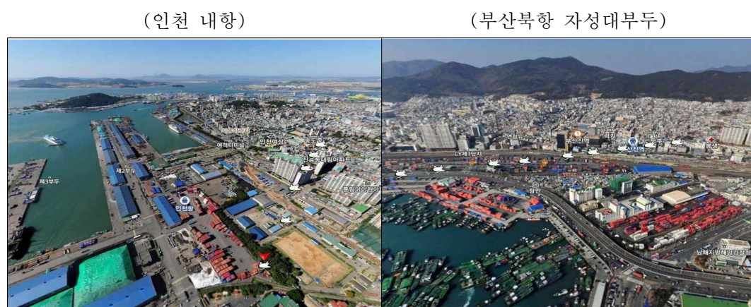
Fig. 2.6 The present status of port redevelopment sites (1)
