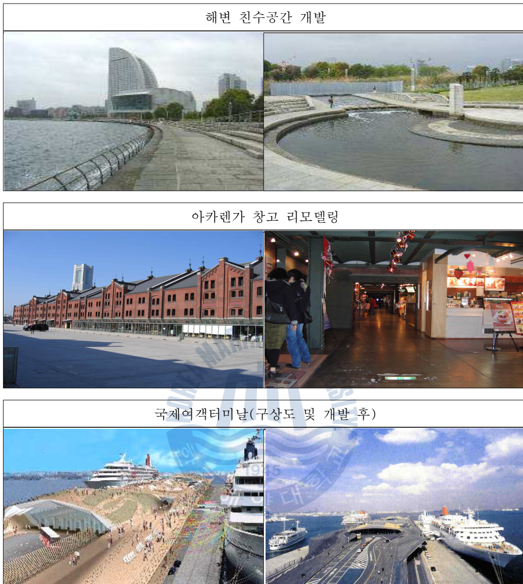
Fig 2.16 Waterfront facilities of Yokohama port
