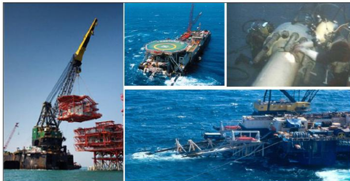
Fig.3.12 Offshore plant and pipeline installation scene [20]
