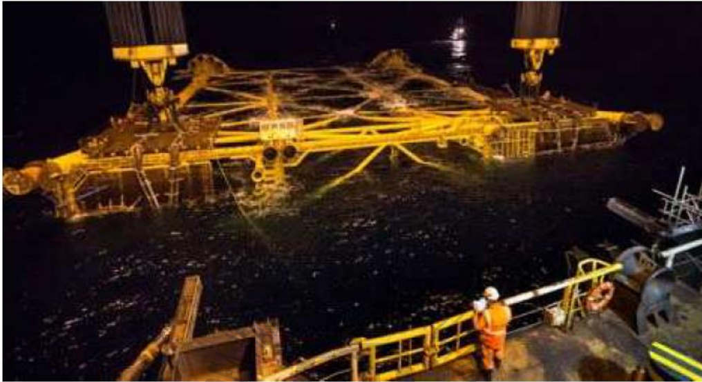
Fig.3.13 Appearance of jacket installed in mariner block [27]
