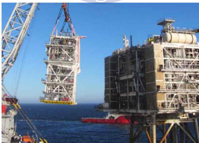
Fig.3.14 Top-side installation of chevron at alder block [28]
