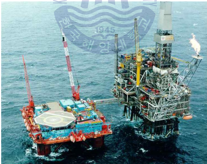
Fig.3.5 Connect offshore accommodations and workshops to telescopic gangway [21]
