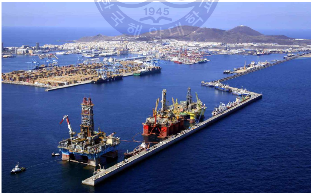
Fig.3.6 View of Las Palmas port in Spain [23]
