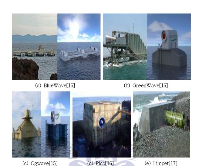
Fig. 1.6 Selected examples of Oscillating water column WECs
