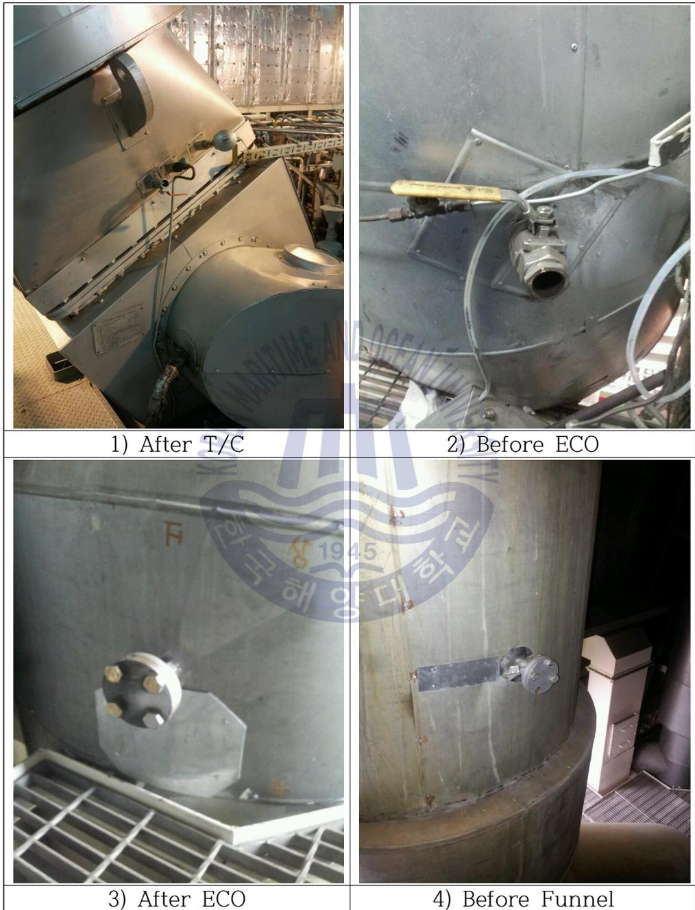
Fig. 2-3 Pictures of sampling locations for soot from 2-stroke engine
