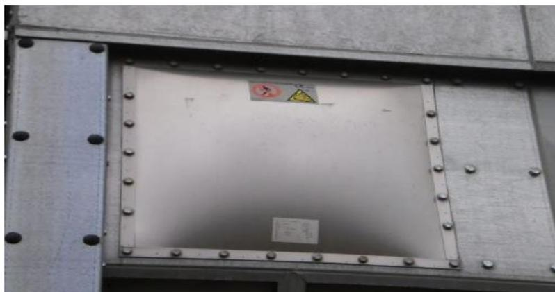
Fig. 4-86 Installation example of an explosion venting panel
