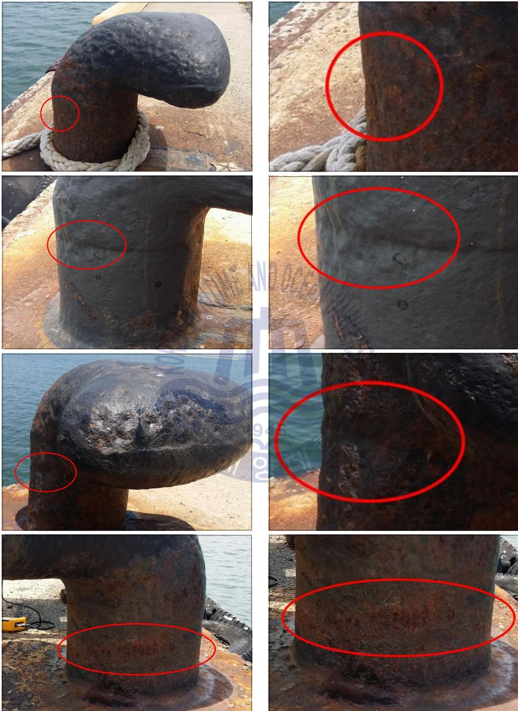
Fig. 28 Measuring position of bollard's thickness
