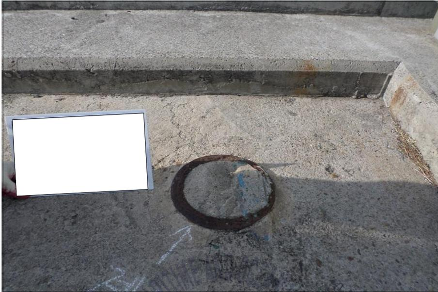
Fig. 23 Case of damaged bollard by broken
