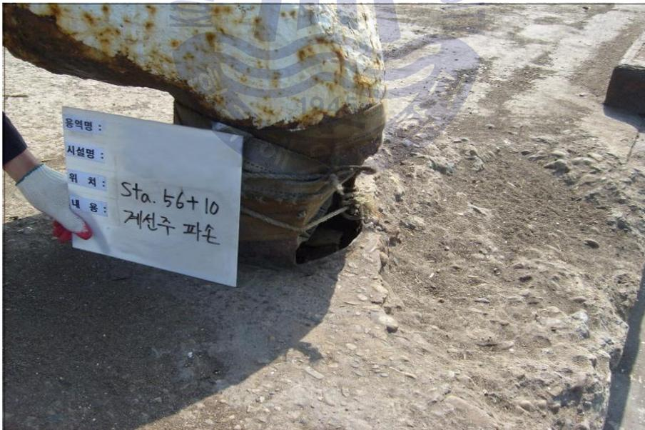
Fig. 22 Case of damaged bollard by fracture
