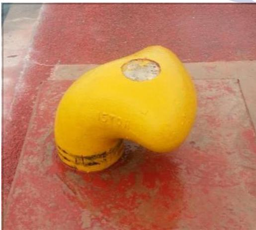
Fig. 2 Bollard (Busan, 15Ton)
