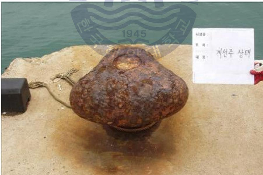
Fig. 20 Case of damaged bollard by corrosion
