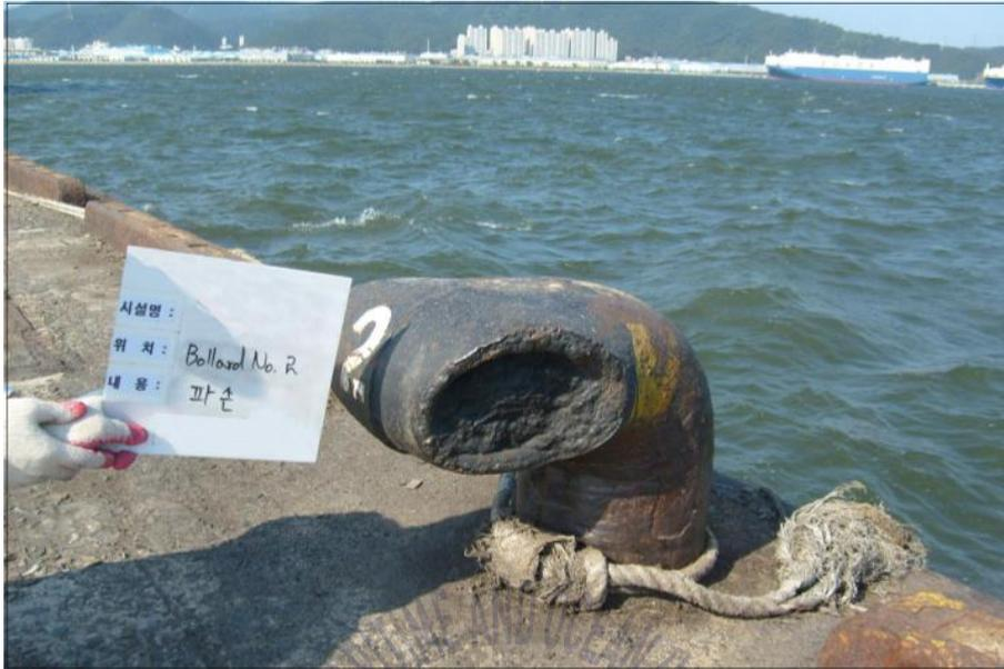
Fig. 21 Case of damaged bollard by fracture
