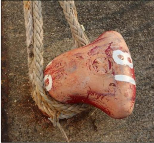
Fig. 4 Bollard (Osaka, 35Ton)
