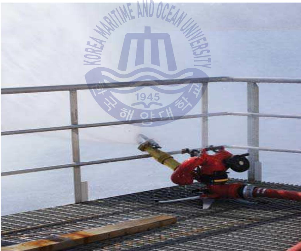
**Fig. 14** Picture of UNITOR's Mobile Water Monitor Spraying
