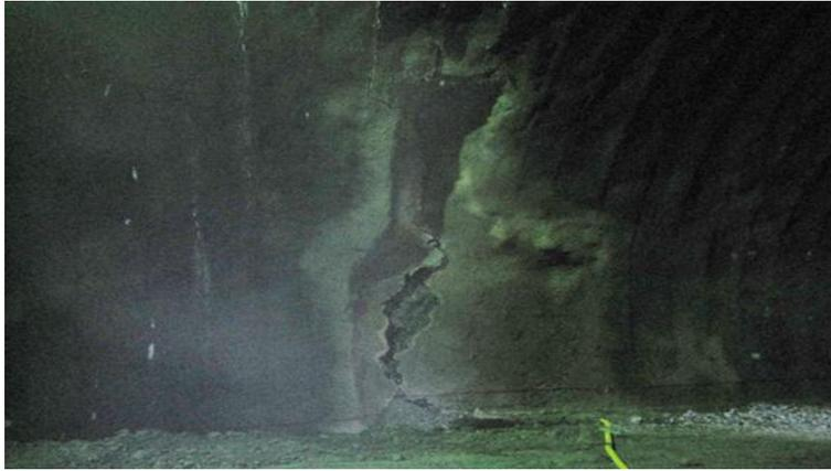
Fig. 3.18 Shotcrete in the sidewall crack and dropout(Volume 0.7m3)
