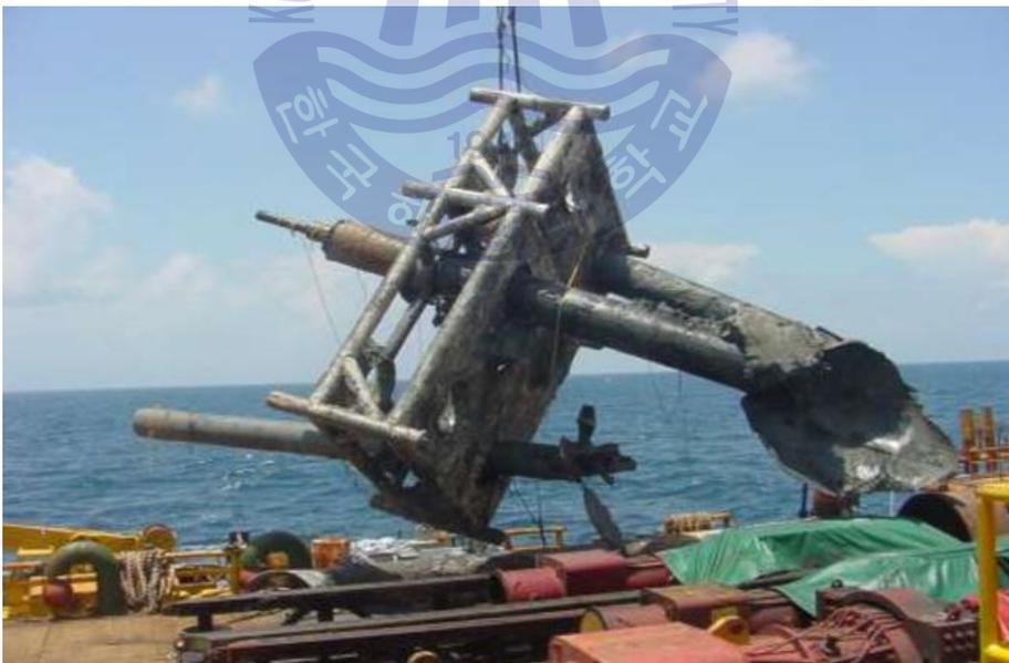
Fig. 8 Template removal by explosives
