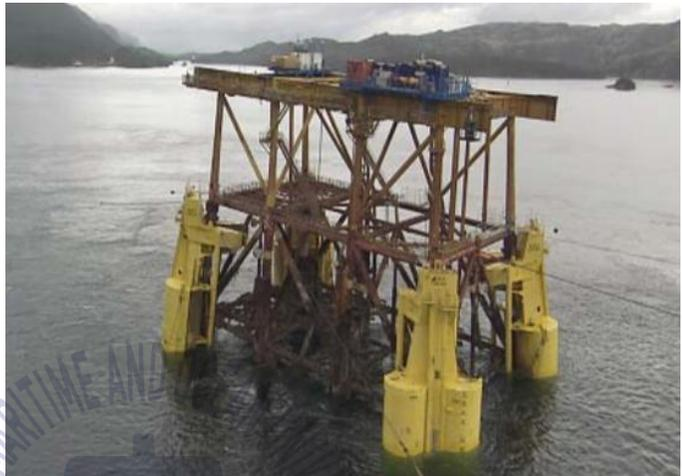
(b) buoyancy tanks attached DP2 jacket
