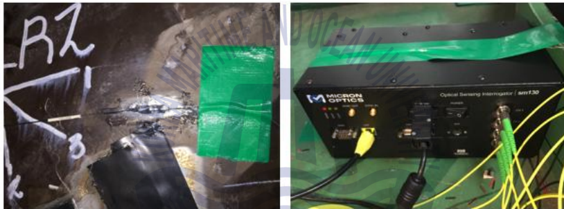
Fig. 3-6 Fiber optic sensor installed on the inner shell plating and the measurement equipment
