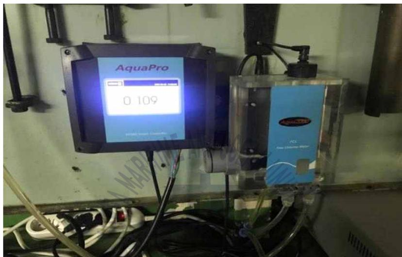
Fig 3.14 Appearance of free chlorine meter
