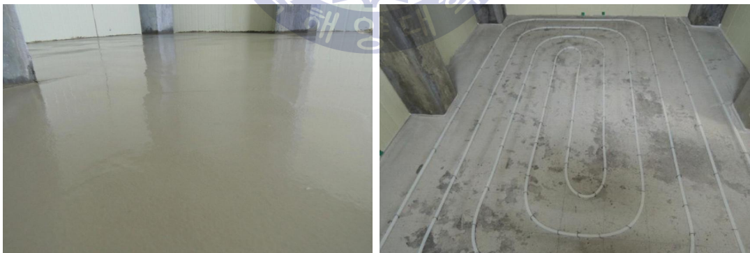
(a) Construction of air-trapped soils
