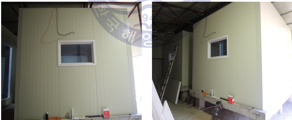
Fig. 3.7 Photograph of buildings constructed for heat storage experiment
