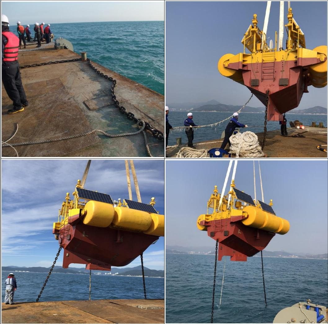
**Fig. 5.21** Mooring line and submerged cable connection and lifting
