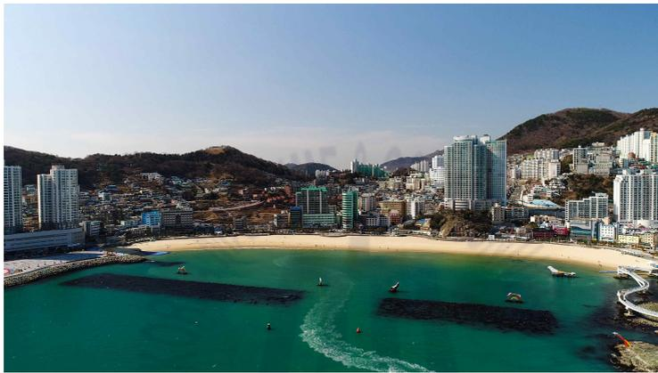
Photo 1.2. Submerged breakwaters to protect beach erosion of Songdo, Busan(<https://www.crowdpic.net>).
