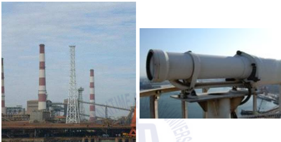
Fig. 8 View of Pohang new port Sector Light
