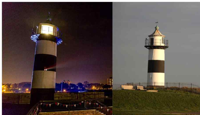
Fig. 25 View of Southsea Castle Lighthouse
