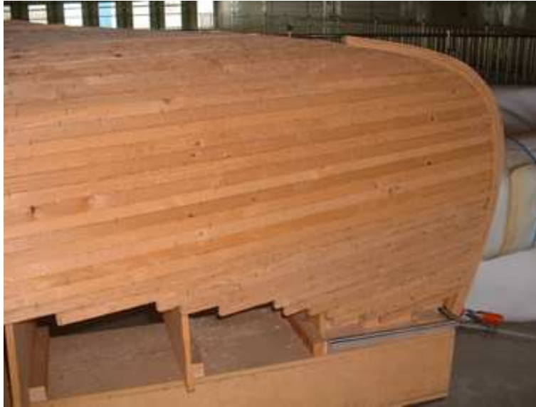
Fig. 13 End of stripping over the strongbacks
