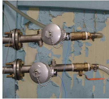
Fig. 5.4 Inlet and outlet of cooling water in heat exchanger
