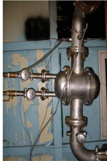
Fig. 5.6 Picture of installed shell & tube and fin-tube heat exchanger
