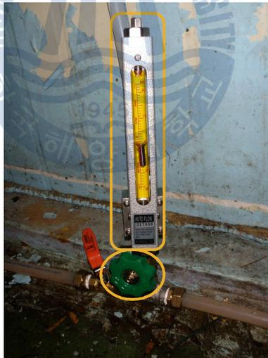
Fig. 4.7 Orifice type flow meter and flow control valve
