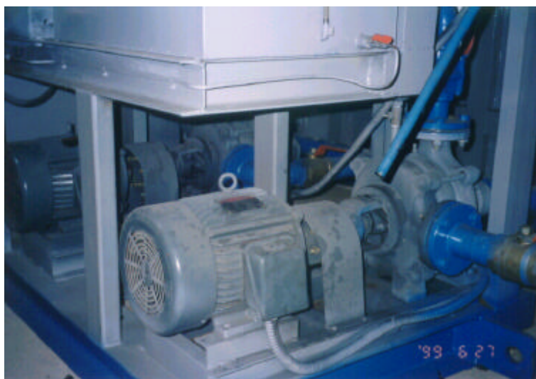
Photo. 2.3 Hot water supplying unit
