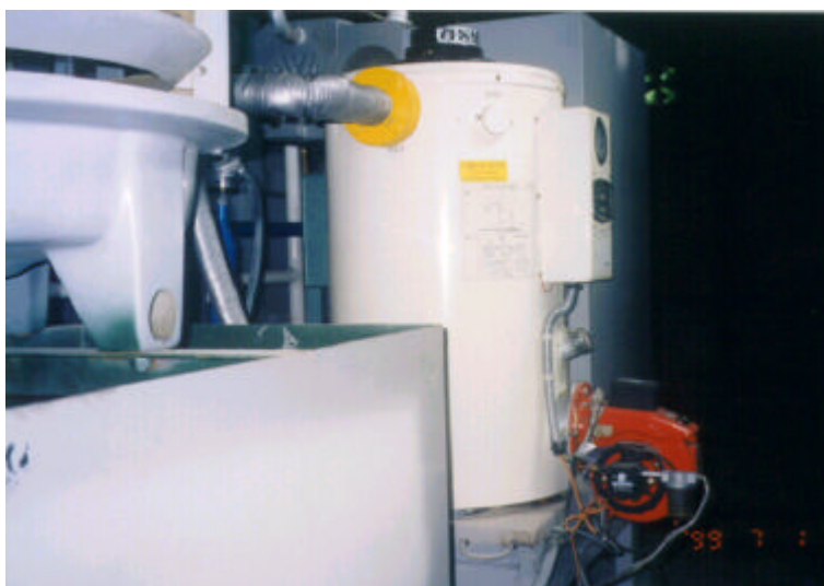
Photo. 2.3 Hot water supplying unit
