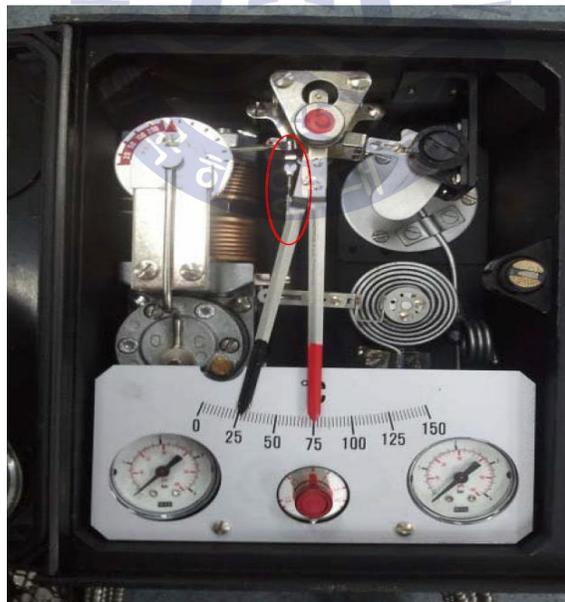
Fig. 4.3 Temperature controller of jacket cooling water cooler (S8243)
