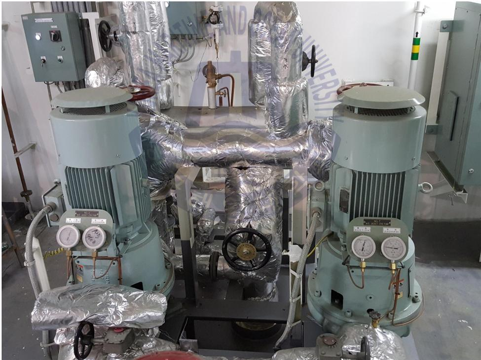
Fig. 2.7 Jacket cooling fresh water pump
