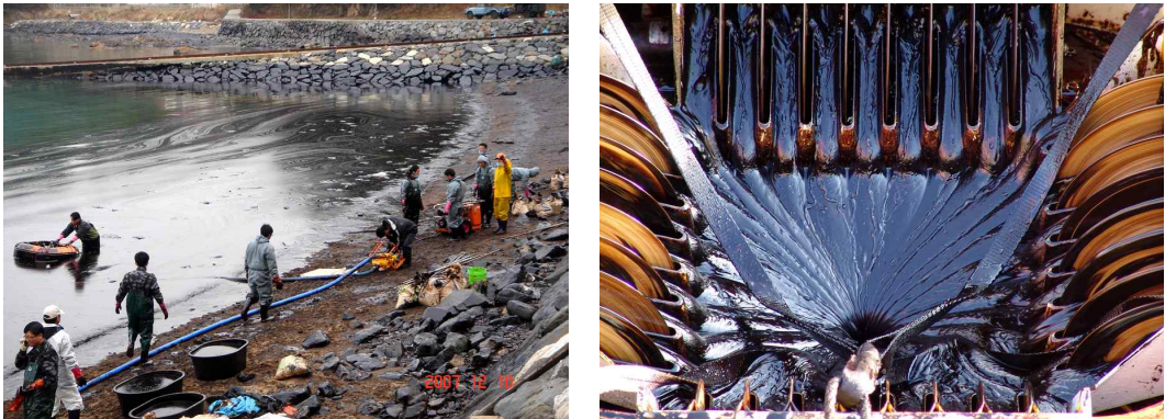
Fig. 2.8 Onshore skimming operations using skimmers
