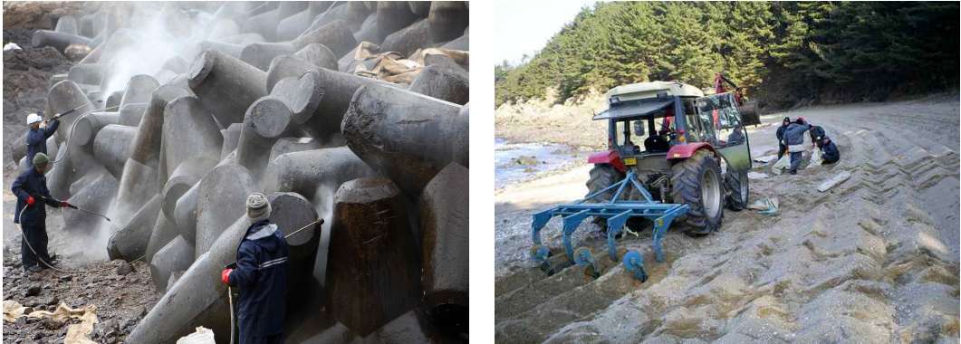
Fig. 2.9 Removal of surface and subsurface oil
