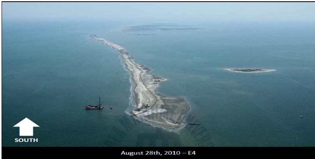
Fig. 4.21 Construction of sand berms for the prevention of shoreline contamination
