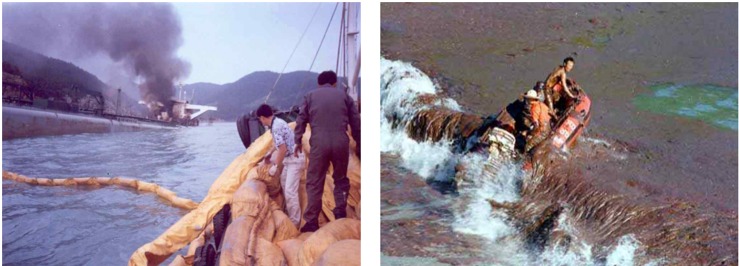
Fig. 2.3 Containment measures for spilt oil at Sea Prince incident
