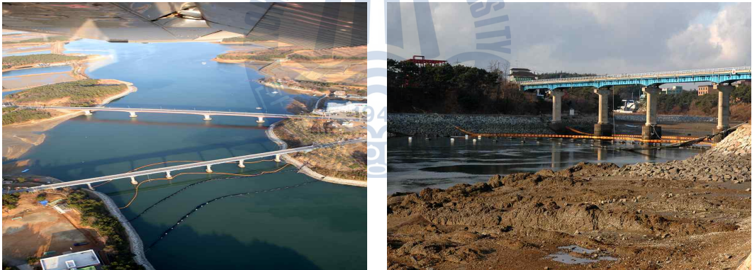
Fig. 2.6 Oil boom deployed for protection of sensitive areas
