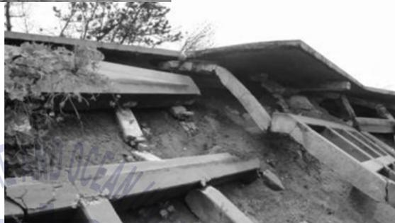
**Fig. 2.4** Levee slope failure due to the overflow(Kim, 2014)
