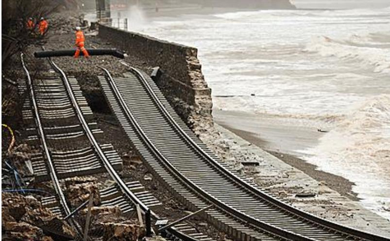
**Fig. 2.6** Levee railroad destruction by typhoon
