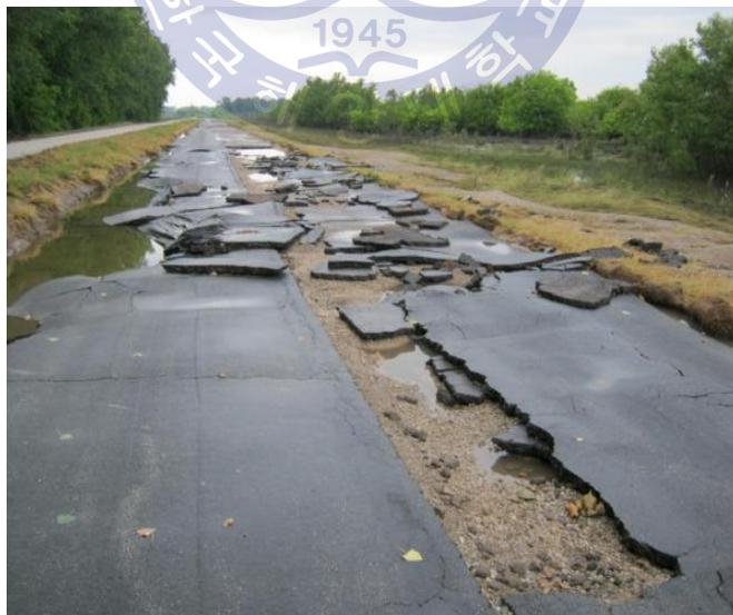
**Fig. 2.5** Missouri river levee road's pavement damage by flood at 2013
