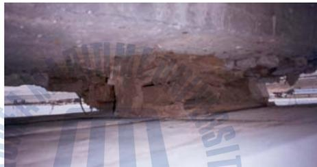
(b) Leakage & bearing deterioration
